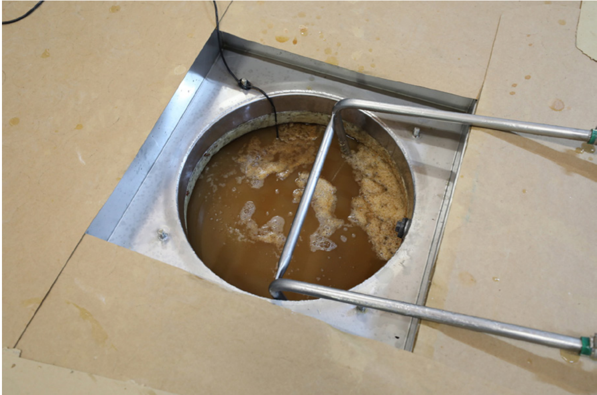
Underground tank for Muscadet fermentation and lees ageing
